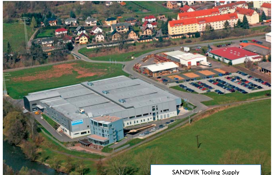
SANDVIK Tooling Supply Schmalkalden: state-of-the-art manufacturing facility on 13,000 m 2 of space.
