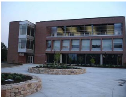
Earl W. Brinkman Manufacturing and Machine Tools Laboratory at the Rochester Institute of Technology, Rochester, NY
