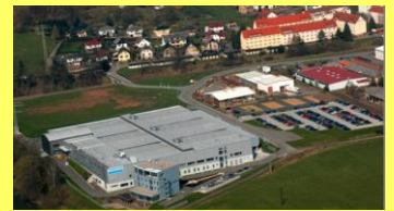
SANDVIK Tooling Supply Schmalkalden: state-of-the-art manufacturing facility on 13,000 m 2 of space.
